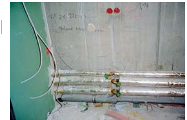
The bathing comfort of the 69 double bed room under construction should not, amongst other things, suffer from sounds of running water. The plastic cuffed JRG Sanipex MT multilayer pipes go far to meeting this requirement.
