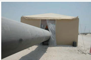
Protecting the welding zone using a tent
