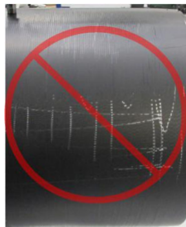
Poor scrape: markings not removed
