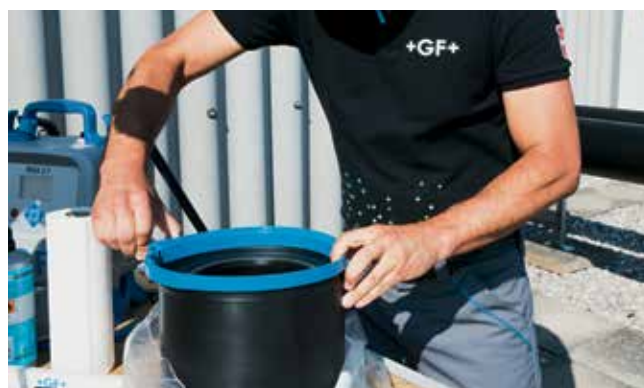
Place the assembly aid on the fitting. Stretch the sealing lip pressing the handles together.
