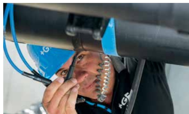
Connect the welding cables to the welding contacts of the fitting and weld according to the instruction manual.
