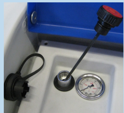
Oil level check & refill
