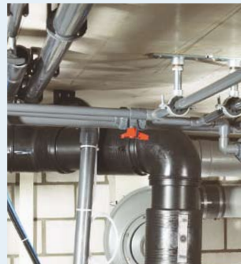
Waste water disposal line for chemicals in CONTAIN-IT Plus or FUSEAL® (PVDF/PP)
