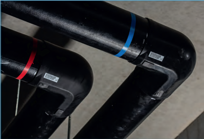
COOL-FIT 2.0 in klimaatapplicatie in winkelcentrum / appartementencomplex
