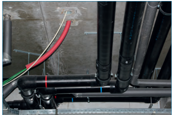
COOL-FIT 2.0 in klimaatapplicatie in winkelcentrum / appartementencomplex
