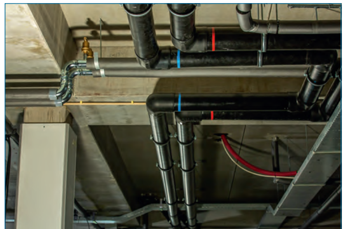
COOL-FIT 2.0 in klimaatapplicatie in winkelcentrum / appartementencomplex
