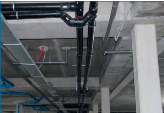
COOL-FIT 2.0 in klimaatapplicatie in winkelcentrum / appartementencomplex
