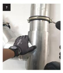
7. Fix Use pipe bracket to secure ecoCOOL onto installation location.
