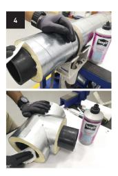
Clean Use lint-free cloth and PE cleaning solution to clean fusion area on both pipe and fitting.
