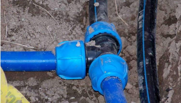
The new pull-out resistant multi-range coupling from GF Piping Systems
