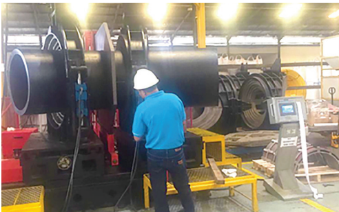
DN1000 Underground Water Supply HDPE - Mining
