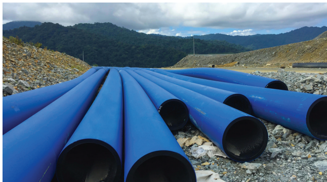
(315mm pipe, water distribution)
