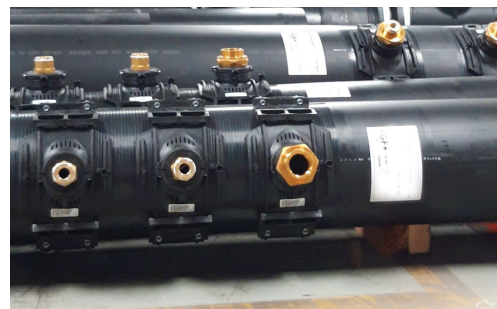
Prefabrication Chiller Plant HDPE - Building Technology
