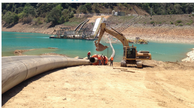
(1000mm pipe, dewatering systems project)
