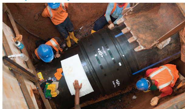
(ELGEF Electrofusion Coupler 1000mm for water treatment project)
