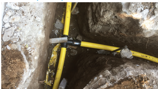
(PE80 pipe & Electrofusion fittings for Gas distribution)
