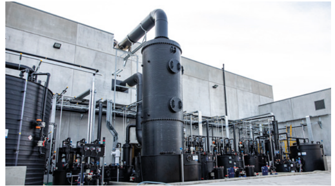
Process instrumentation as well as manual and automated valves streamline the operation of the scrubber park.
