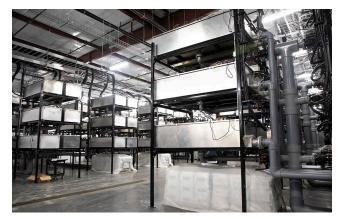
Rhodium uses immersion cooling, fully submerging their servers to achieve maximum efficiency.
