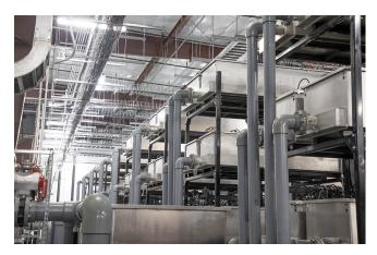
ChlorFIT, made with Corzan® CPVC, is a highly robust and corrosion resistant Schedule 80 piping system offering superior reliability and long-lasting performance in commercial and industrial applications.
