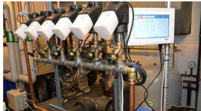
Sensors/valves have been installed on each hot water routing at Orkerød Nursing Home, shown here in the control room. On the right is the touch screen for the system.
