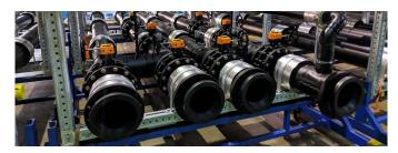
Prefabricated pipe modules ready to be shipped to the construction site.
