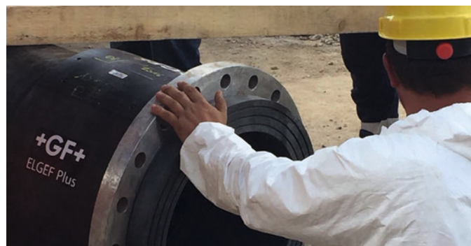
Perfect and easy fit for PE repairs: ELGEF Plus coupler and GF Piping Systems flange d500 mm.
