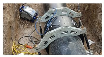
Simple and reliable: The ELGEF Plus electric welding system matches welding machine, tools and fittings to one another.
