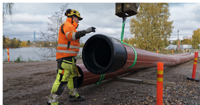
Easy and fast installation of the ELGEF Plus electrofusion coupler.
