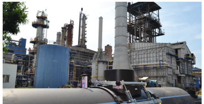
Fast onsite integration of a d1000 mm ELGEF Plus saddle with a d500 mm outlet.
