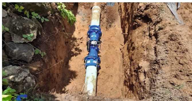
For advanced pressure control the NeoFlow was installed in two pressure supply zones.
