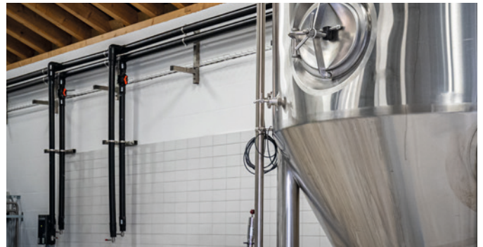
The two master brewers were able to cut the already pre-insulated plastic pipes and install them in a single session as desired without any previous expertise.
