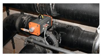
New Butterfly Valve 565 in the filter system
