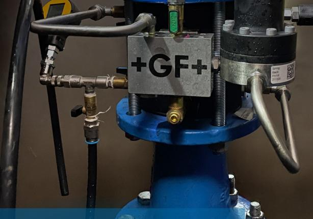
Largest water utility in Slovakia has installed NeoFlow, the pressure regulating valve (PRV) by GF Piping Systems to reduce the water pressure in critical points throughout a village.
