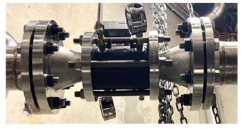
Thanks to a reduction from DN100 to DN50, a far more lightweight and compact NeoFlow PRV could be installed at Pearlwater.
