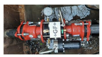
Thanks to its axial flow construction, NeoFlow ensures a stable flow from 1% to 100% opening, even at a small operating differential.
