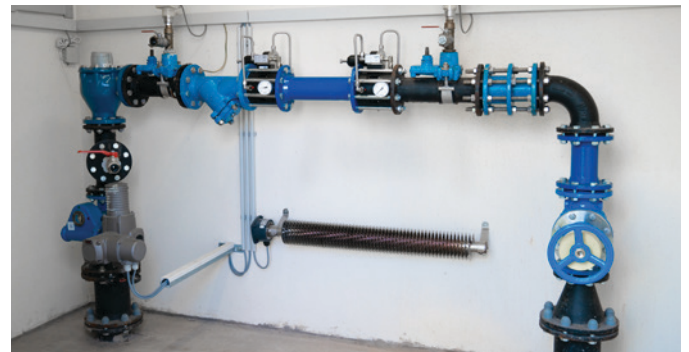
Due to its simple construction without an actuator stem and diaphragm, NeoFlow has a long service life and requires little maintenance.
