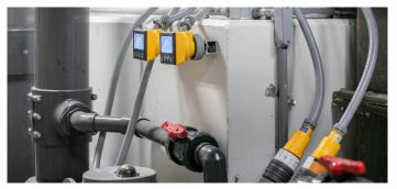
Water enters the exhibits after deaeration. The ORP probes are installed in-line using wet-tap devices, so they can be pulled for maintenance without getting wet or shutting anything down.
