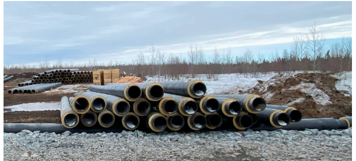
The Tataskweyak Cree Nation enhanced its drinking water system with GF Urecon's solution, installing over 25,000 feet of insulated HDPE pipe to deliver raw water to a new treatment facility.
