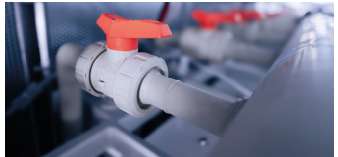
The installation of 84 ball valves allows for the convenient isolation of the distribution or collection pipes from the system, facilitating peace of mind for tests and maintenance.
