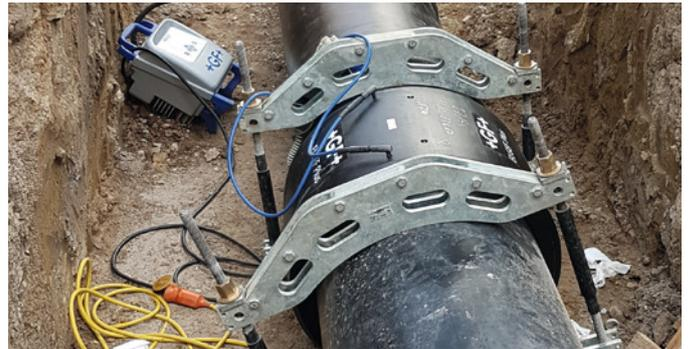
Simple and reliable: The ELGEF Plus electric welding system matches welding machine, tools and fittings to one another.
