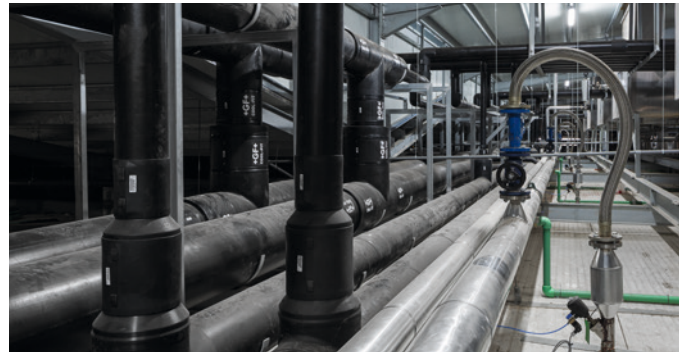
Almost 2.000 meters of COOL-FIT pipe was installed at Champinter.
