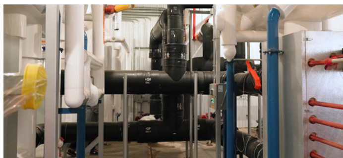
Safe, lightweight and quick to install, COOL-FIT 4.0 lowers structural demands on buildings and supporting structures while reducing the need for heavy and expensive transport aids.
