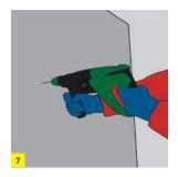
Drill the marked points with a driller and place dowels into the holes.
