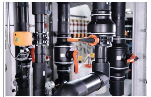
An installation of the pre-insulated COOL-FIT piping system.
