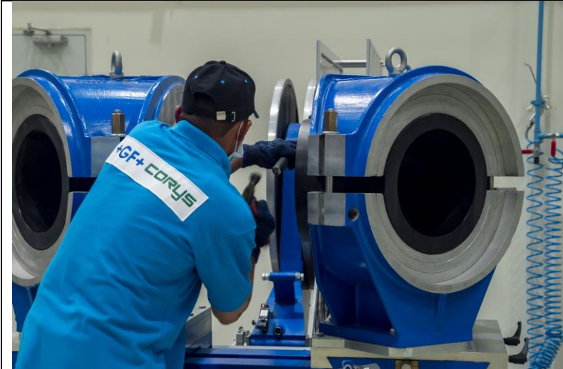
Working in the GF Piping Systems' new prefabrication site in Abu Dhabi.
