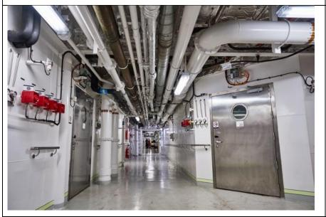
Around five kilometers of thermoplastic pipes are installed on the ship.
