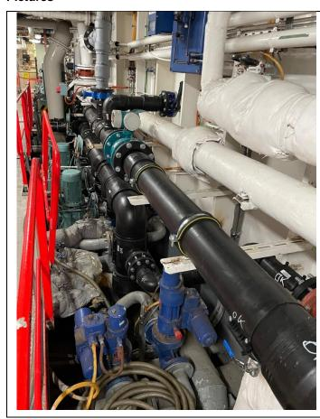
Thanks to the material properties of the ecoFIT and INSTAFLEX piping systems, the hot and cold water manifold benefit from a corrosion- and maintenance-free operation.
