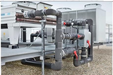
Leitwerk AG selected a fully pre-insulated plastic piping solution to increase reliability and improve energy efficiency by up to 25%.
