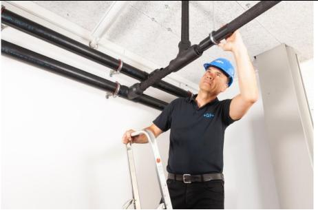
The COOL-FIT 2.0 Push System offers an easy plug-and-play installation thanks to mechanical connections, bendable pipes, and modular adapter technology.
