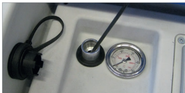
Oil level check & refill
