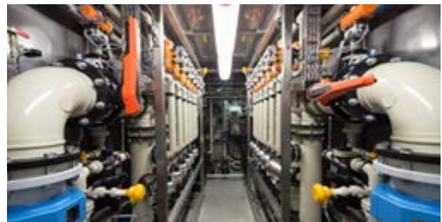
Redundant ultrafiltration module with GF piping, valves and instrumentation.
