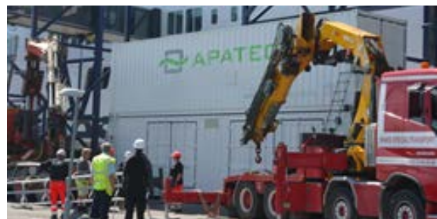
Containnerized MarinePaq onshore installation at the port in Denmark.
