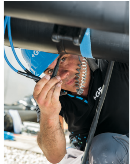
Easy and safe welding on site: Without hazardous vapors, smoke and flame formation.
