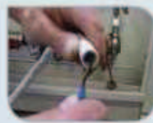
9 Fit the pipe to the manifold
