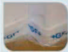
1 Install edge insulation strip
