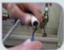
8 Fit the pipe to the manifold
