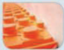
2 Lay insulation panel
