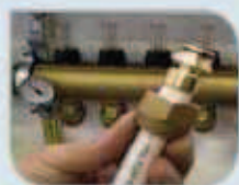
9 Insert the pipe into the fitting
