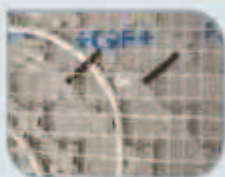
8 Lay anti-shrinkage mesh
