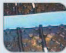
5 Position exp. joint profile
