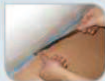
13 Use flanking strip to isolate the acoustic floor from the wall and skirting board
