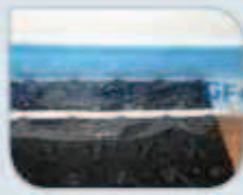
2 Lay insulation panel
