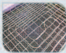
8 Lay anti-shrinkage mesh
