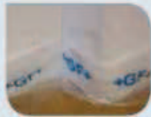
1 Install edge insulation strip
