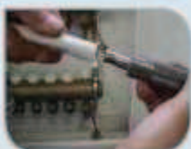
7 Let pipe pass through the wall
