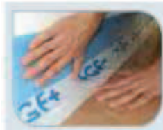
1 Install edge insulation strip
