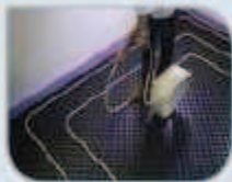
5 Lay the pipe
