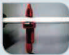
9 Fit the pipe to the manifold
