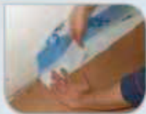
3 Lay insulation panel
