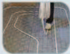
4 Lay the pipe
