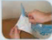
1 Install edge insulation strip
