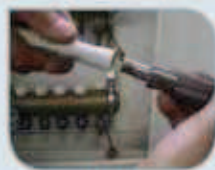
8 Fit the pipe to the manifold
