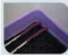
6 Let pipe pass through the wall
