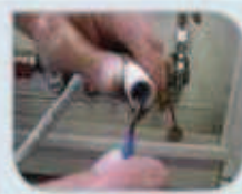
9 Fit the pipe to the manifold
