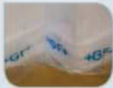
1 Install edge insulation strip
