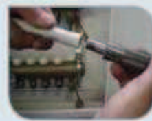
6 Let pipe pass through the wall
