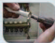
6 Let pipe pass through the wall
