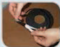
13 Use flanking strip to isolate the acoustic floor from the wall and skirting board
