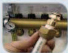
10 Insert the pipe into the fitting
