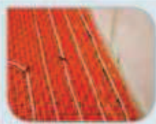
8 Lay anti-shrinkage mesh
