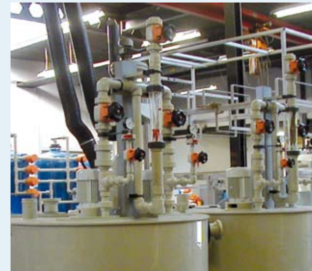
Chemical Drainage and Waste Water Treatment in PROGEF Standard, PVC-U, PE, FUSEAL
