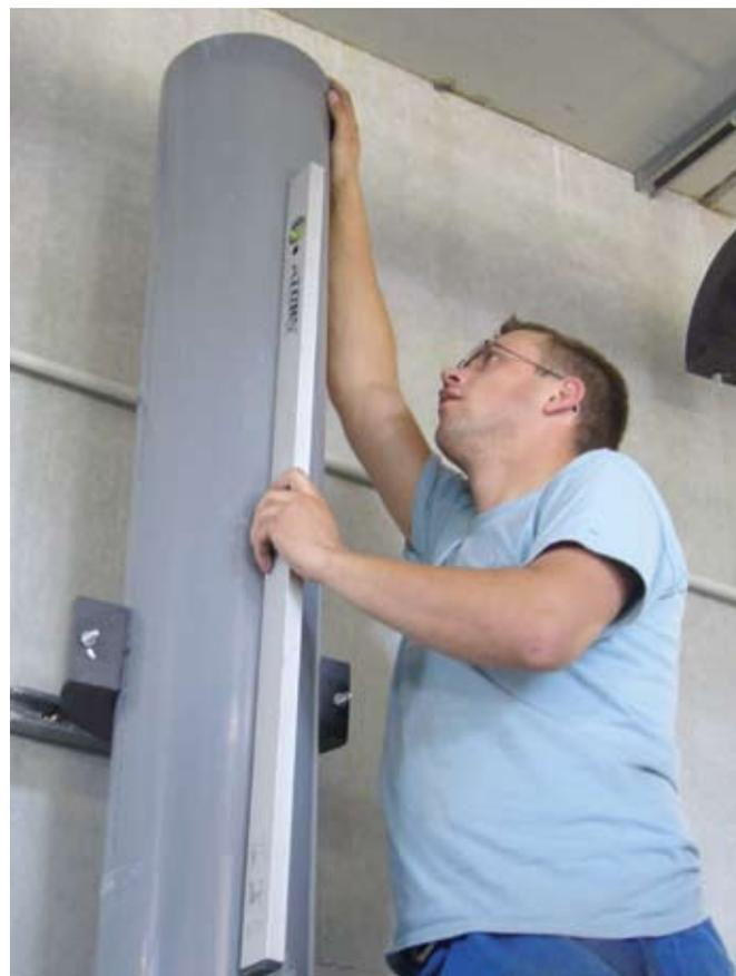
store such as this presents a challenge. The installers were trained by GF in advance on how to work with a pre-insulated plastic pipe system. Well-trained professionals are the guarantee for a smooth installation process and top quality system. COOL-FIT ABS Plus installations are based on the time-tested and proven solvent cement joining method and are easy and safe to install with no expensive equipment required.
