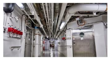
Around five kilometers of thermoplastic pipes are installed on the Global Mercy.
