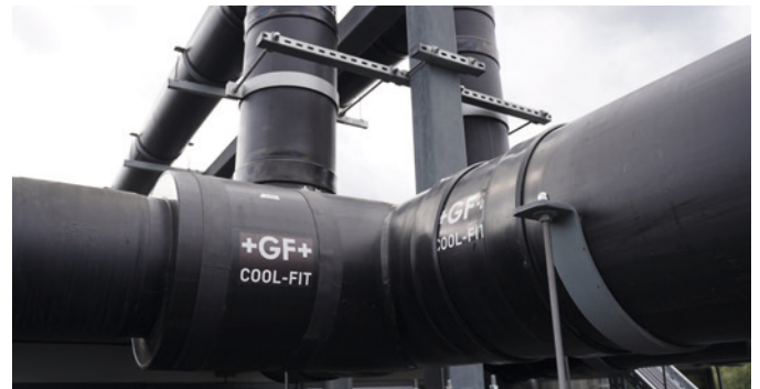
The lightweight, largely prefabricated pipe system was easily assembled and reliably joined by electrofusion within a few minutes.
