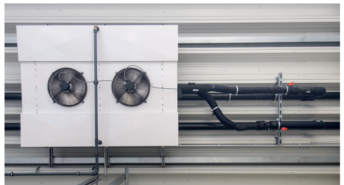
The connection to the circulating air coolers with COOL-FIT 2.0.
