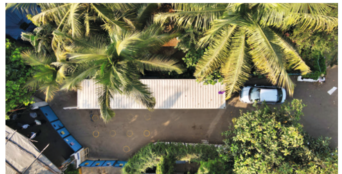
Mobile water treatment in containers thanks to process automation.
